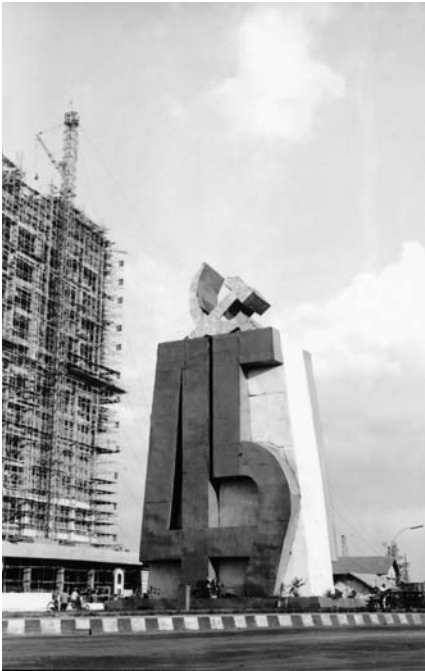
7. Monument with traditional communist symbols hammer and sickle for the 45th anniversary of the PKI. On the left the PKI head-office under construction: "In the Spirit of the Red Banteng".
